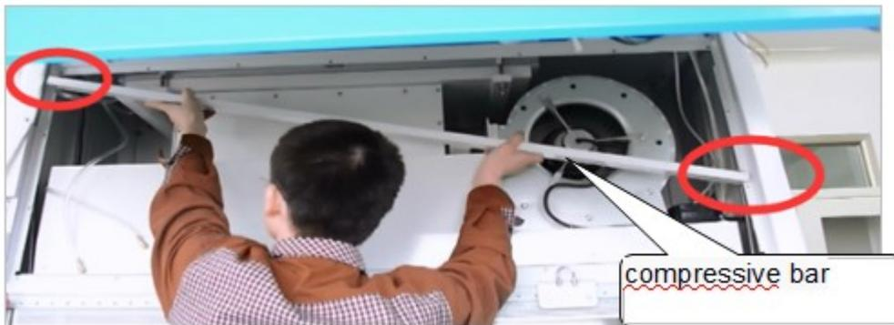
e) Remove internal front panel, pull out the ducts, record the position.
