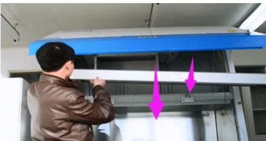
r) Install the fan installation board, reconnect ducts.
