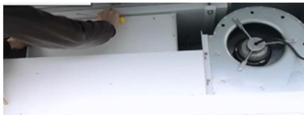
v) Install press bars, tighten nuts.
