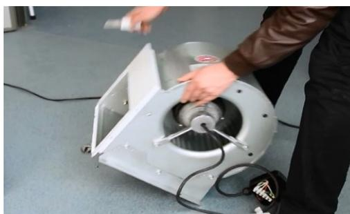
n) Replace the same type of fan, install fan mounting plate connector and gluing.
